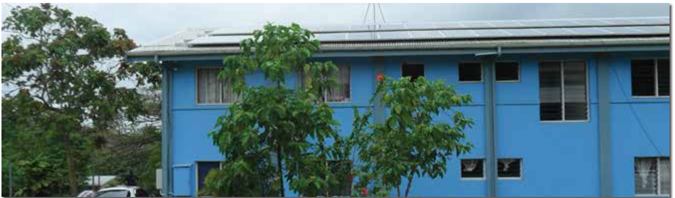
The 10kW array on the Sanma Council offices, Espiritu Santo, Vanuatu
